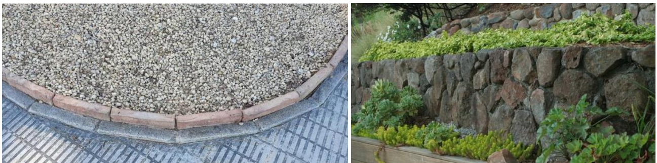
EFFICIENT CONTAINMENT SYSTEMS AGAINST RUNOFF
